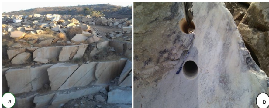
Figure 3. Marble quarry wastes, due to improper mining and drilling activities respectively.
