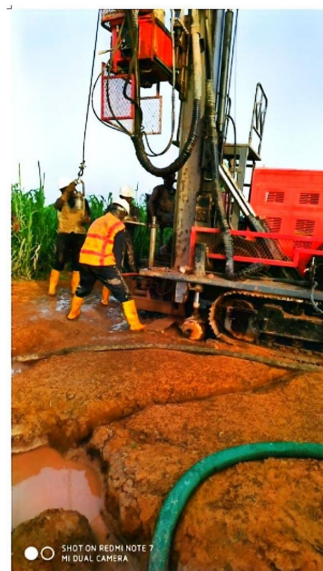
Figure 3. HYDX-5A Multipurpose core drilling rig.
