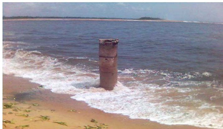
Figure 14. Well exposed at the mouth (May 2007).
