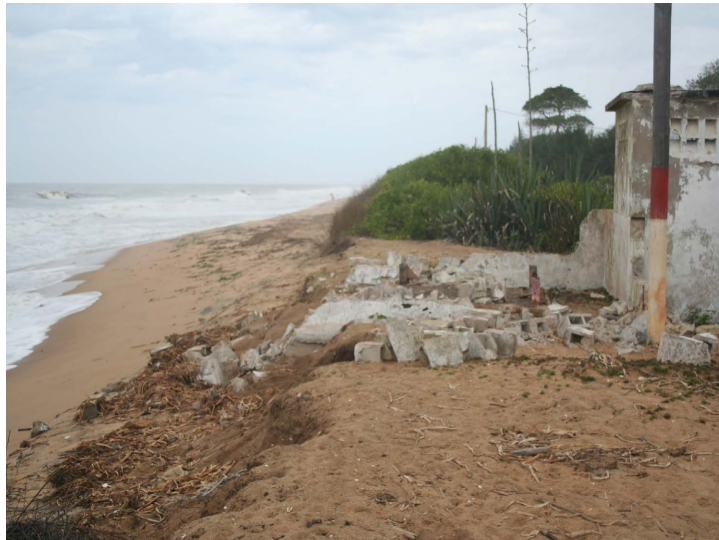
Figure 12. Erosion slope 50 m from.
