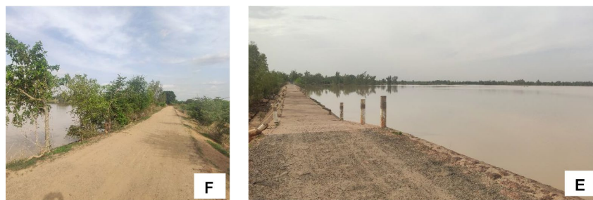
Figure 2. Site of Gonsé dam. (A) Location; (B) The dam site during the rainy season (Google Earth image, September 2023); (C) The site during the dry season (Google Earth image, March 2023); (D) Geophysical exploration area; (E) View of the lake and concrete spillway; (F), view of the southern section of the earthen embankment.
