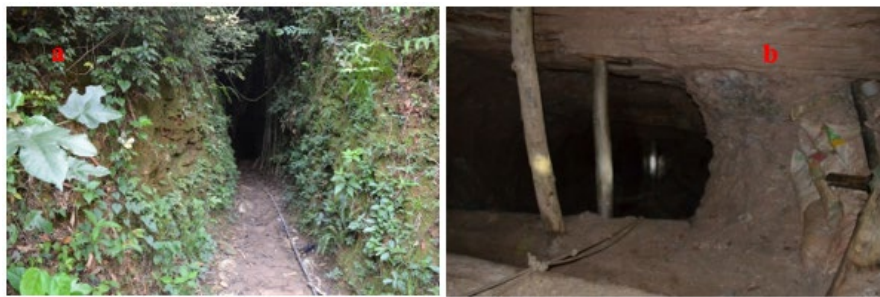
Figure 4. (a) An underground adit; (b) Room and pillar mining with timber supports.
