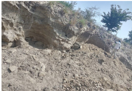
Photo 6. Destruction of yards and landslides in Alhèridè streams, December 2023, Kazaboua river border.
