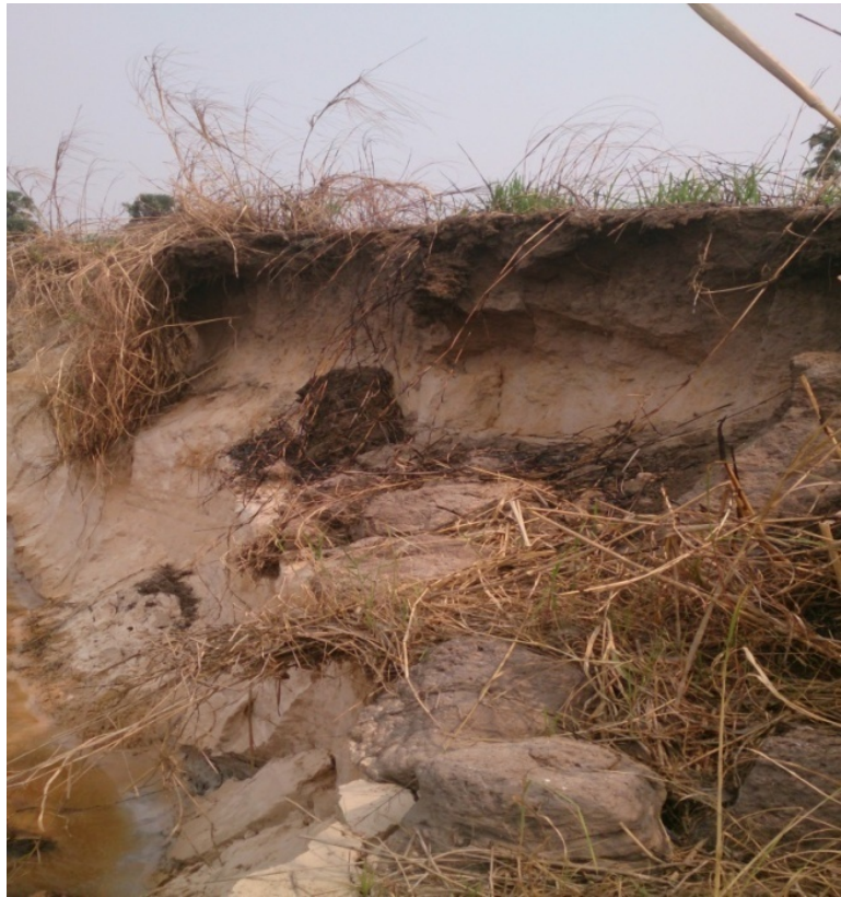
Figure 6. Collapse of sandy riverbanks.
