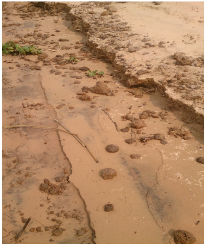
Figure 5. Surface erosion due to wave action.
