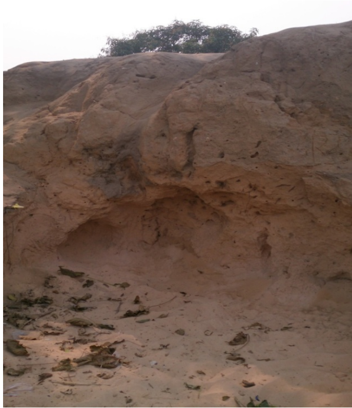
Figure 4. Escapement at the foot of the riverbank in a clay soil.
