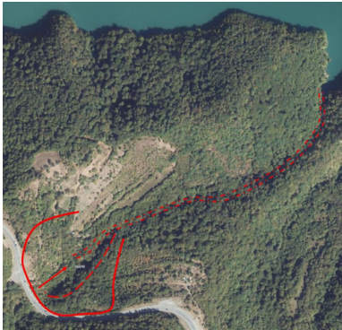
Figure 5. Top view of landslide #4.
