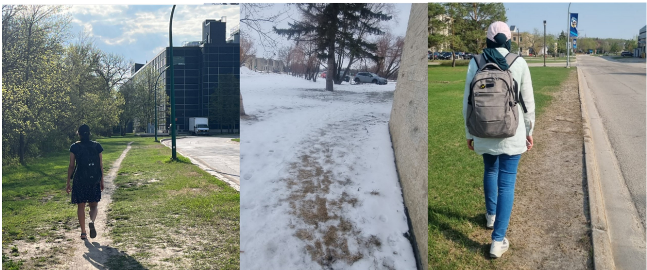
Figure 5. The missing sidewalks at different buildings on the University of Manitoba's Fort Gary Campus. (Left: Wallace building. Middle: Sinnott Building in St. Paul College. Right: Max Bell Center on Sidney Smith St. Source: author).
