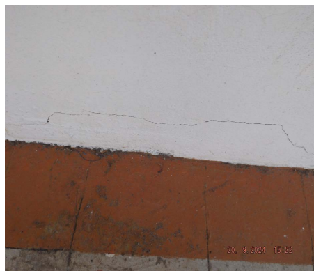
Figure 7. Horizontal crack emanating from a door frame.
