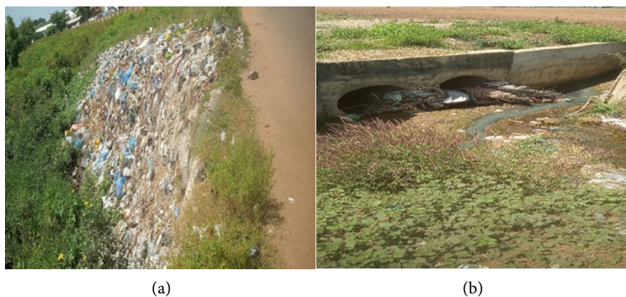
Figure 6. Disposal of SW in open space (a) and a choked drain (b).
