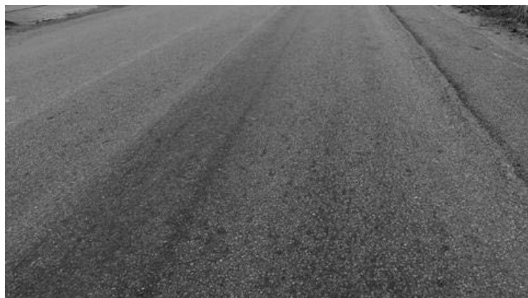
Figure 4. Image of rut converted to grayscale with the BGR2_GRAY filter.
