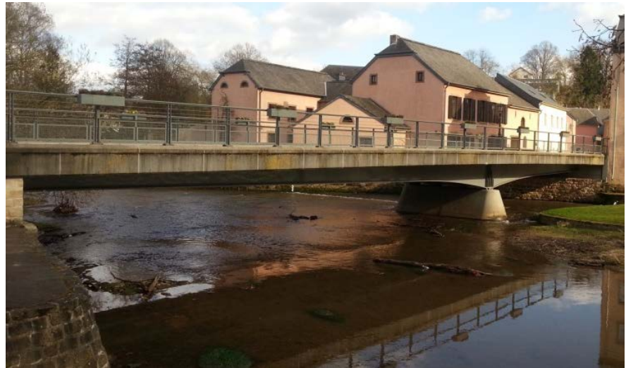
Figure 15. Bridge in Useldange in spring 2015.
