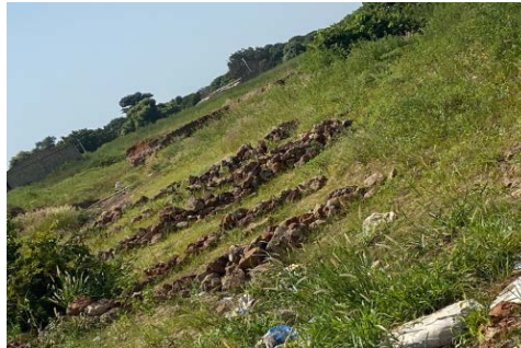
Figure 9. Rows of rocks to reduce wave pressure.
