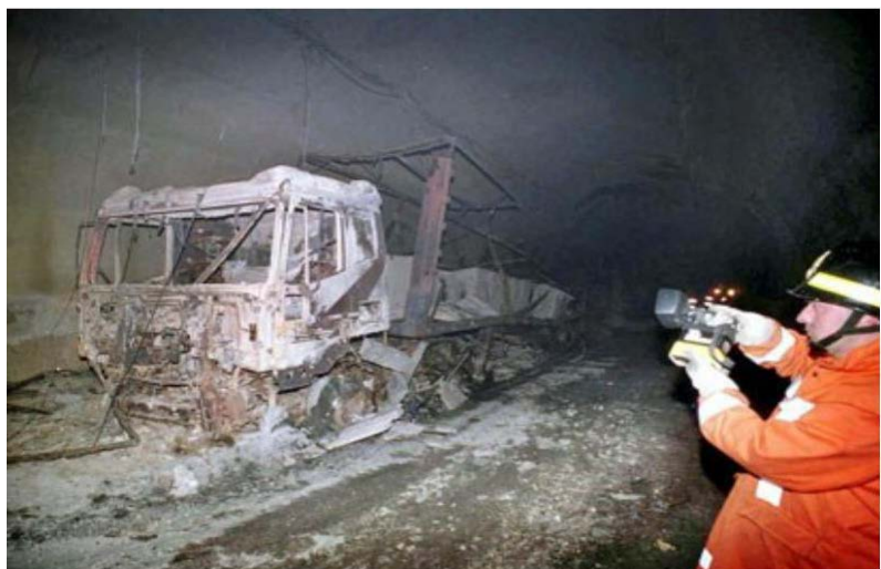
Figure 16. A scene after the 1999 fire in Mont Blanc tunnel (Wallis, 2021).
