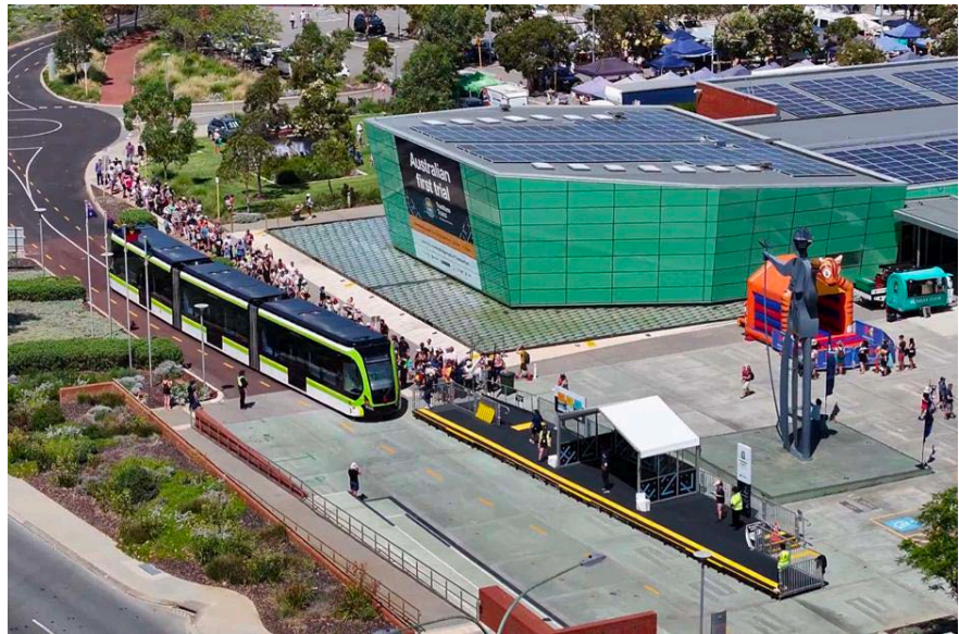
Figure 4. The trackless tram trial and the community open day at city of Stirling, Perth, in October, 2024, with the first Chinese trackless tram in Australia.
