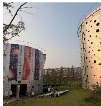
Figure 5. Exterior view of Xiaohe park.
