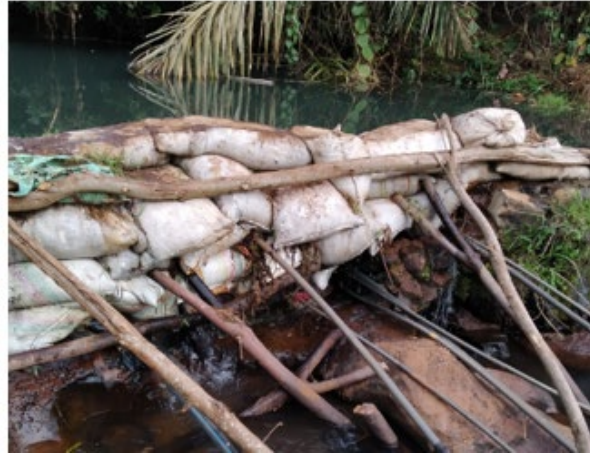
Figure 3. Dikes built for water catchment on Meloung stream.
