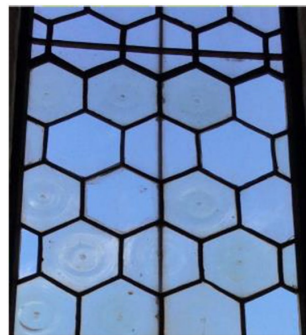
Figure 28. Rests of blown-glass hexagon 14th century glass next to replaced modern glass.
