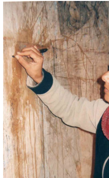
Figure 16. Mechanical cleaning of egg waste (Bengül, 2005).
