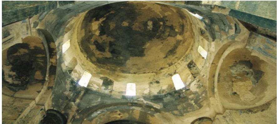
Figure 3. Dirty traces of streams in the dome (Bengül, 2005).
