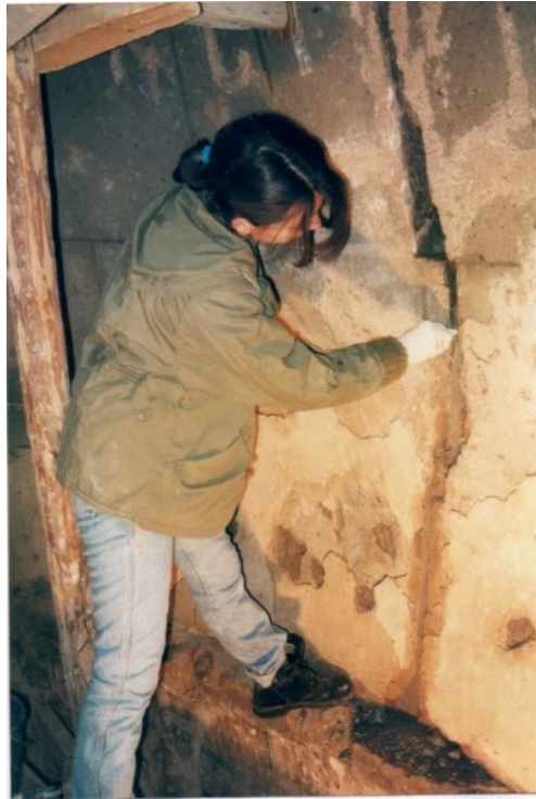
Figure 21. Filling process of the deep cracks (Bengül, 2005).
