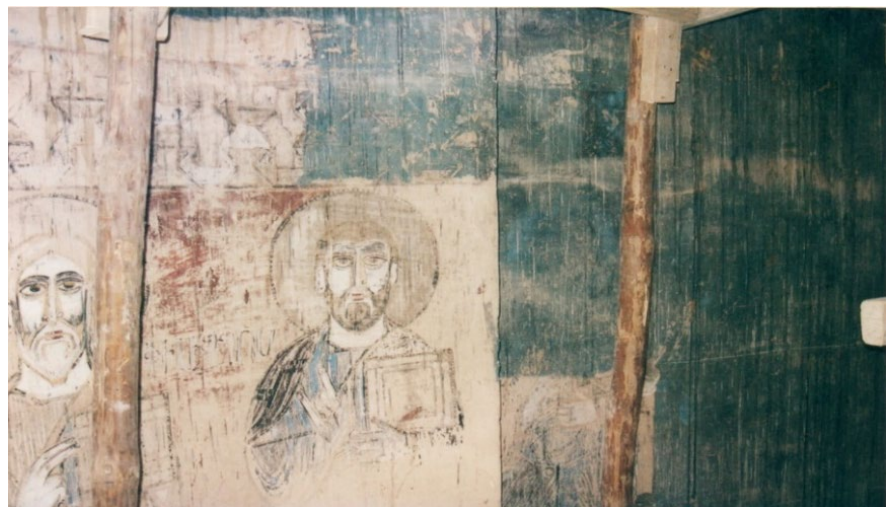
Figure 22. The blue paint applied in the form of whitewash on the apse (Bengül, 2005).
