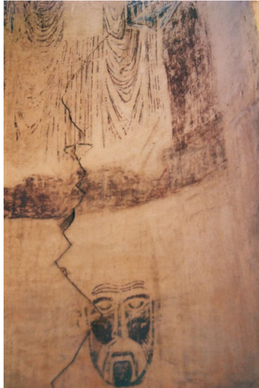
Figure 20. Vertically descending zigzag crack (Bengül, 2005).
