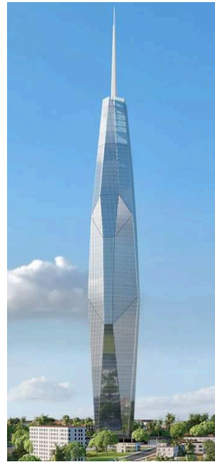
Figure 3. The construction project of Tower F.
