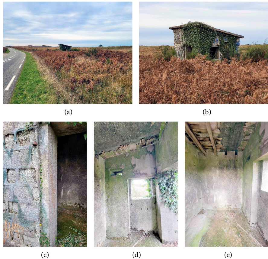
Figure 5. Roc'h Trévél station— 3.5 \times 3.5 emplacement 5—(a) vision from the access road entrance; (b) South-East vision; (c) parallel rows made by concrete blocks and local stones at the entrance; (d) interior East side: square window aperture and rectangular aperture; (e) ceiling: portions of the formwork wood panels, wood supports and concrete portions.
