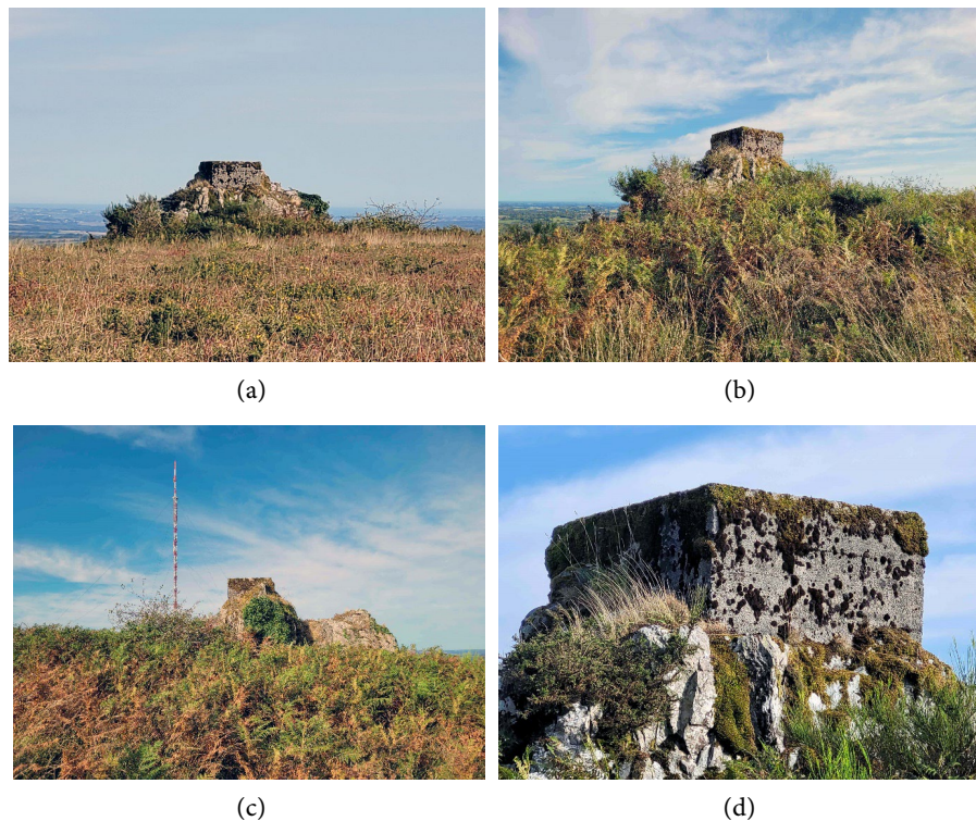
Figure 5. Y8— Wotan II turntable concrete basement 7—(a) view towards the north; (b) view towards the north-west; (c) view towards the west, in the background, antenna of the TV Relay Emitter of Roc'h Trédudon; (d) turntable concrete basement, detailed view.
