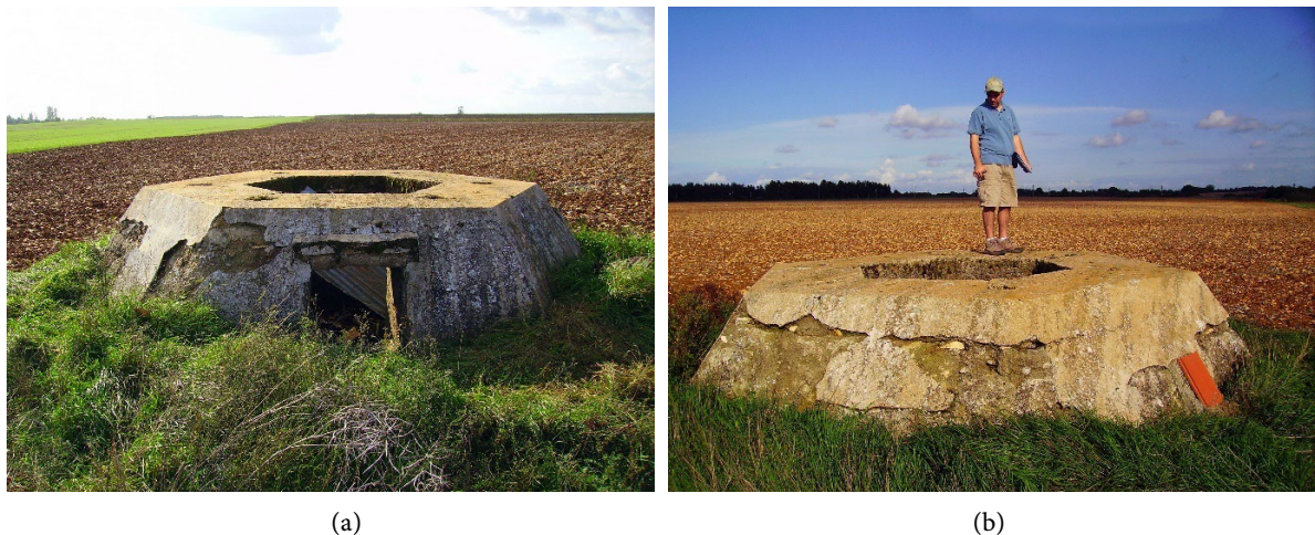
Figure 6. V229 emplacement (6)—(a) North vision with fixation holes for the radar base and square inspection opening; (b) South vision.
