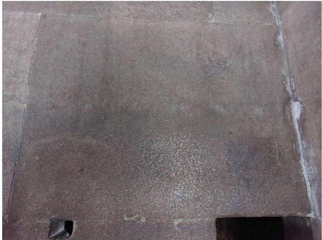
Figure 1. The granite lintel of the north wall over the entry into the Upper Chamber inside the Great Pyramid. The northern shaft (left) begins 2.48 meters from the east wall (right). Photo from 2021.
