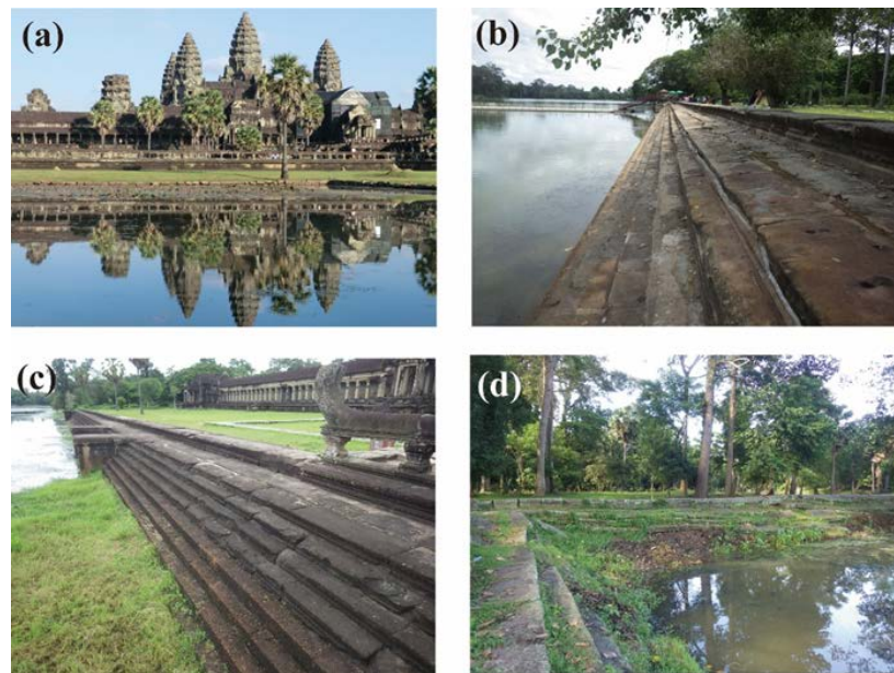
Figure 1. Photographs of the Angkor Wat temple. (a) The main structure inside the surrounding wall of the Angkor Wat temple, (b) the central part of the outer revetment of the western surrounding moat built of the gray to yellowish-brown sandstone blocks (the upper part) and laterite blocks (the lower part), (c) the central part of the inner revetment of the western surrounding moat built of the gray to yellowish-brown sandstone blocks (the upper part) and laterite blocks (the lower part), and (d) the northwestern corner of the outer revetment of the surrounding moat in better preserved condition than elsewhere.
