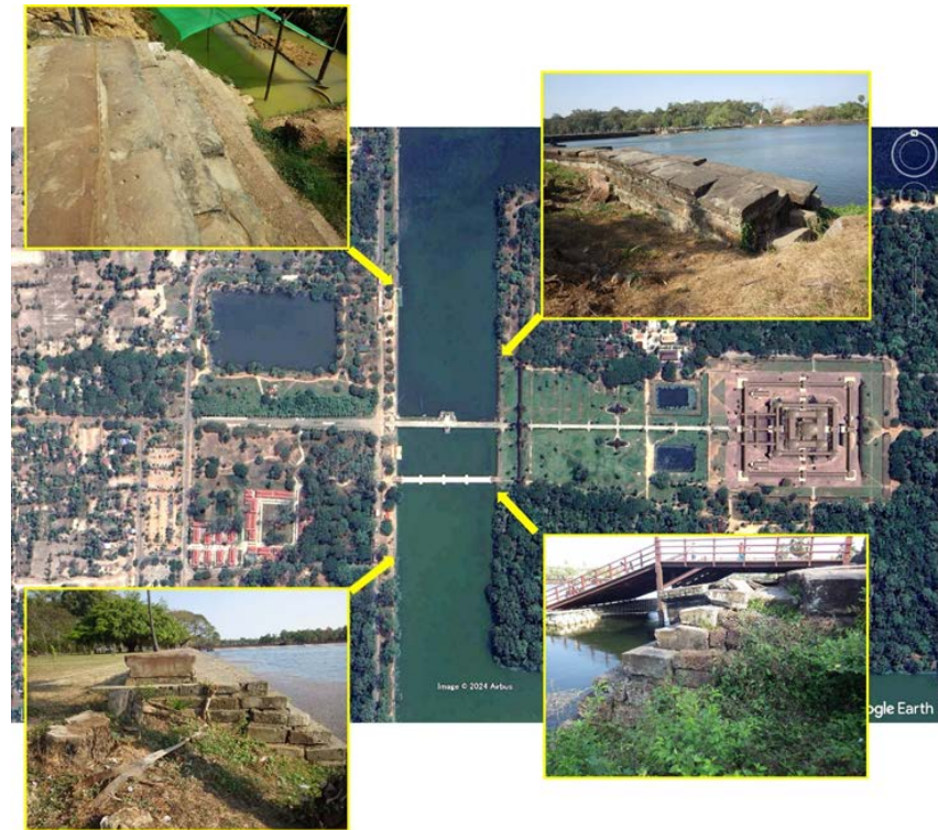
Figure 5. Photographs of the central revetment of the western surrounding moat at the Angkor Wat temple, showing the end faces of the western central part of the revetment of the surrounding moat built of the gray to yellowish-brown sandstone blocks. There is a clear boundary between the outer and inner revetment in the central part of the western surrounding moat and the rest of the revetment.
