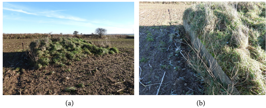
Figure 11. Bunker or platform 9. (a) Vision towards West; (b) uncovered concrete South side.
