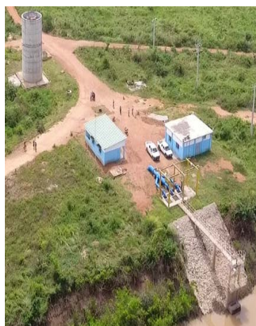
Figure 3. First water pumping station in the irrigated area of M’Bahiakro [19].
