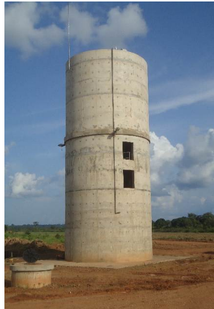
Figure 4. M'Bahiakro rice-growing perimeter regulation reservoir.
